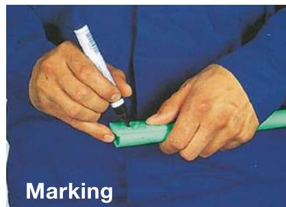
3. Mark the required depth of pipe insertion into the fitting (for a given outer pipe diameter - see the table).
