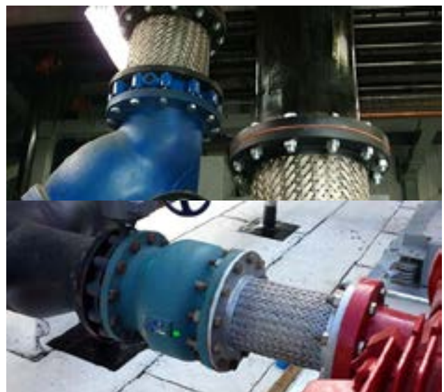
PUMPS WITH FLEXIBLE CONNECTORS IN USE
